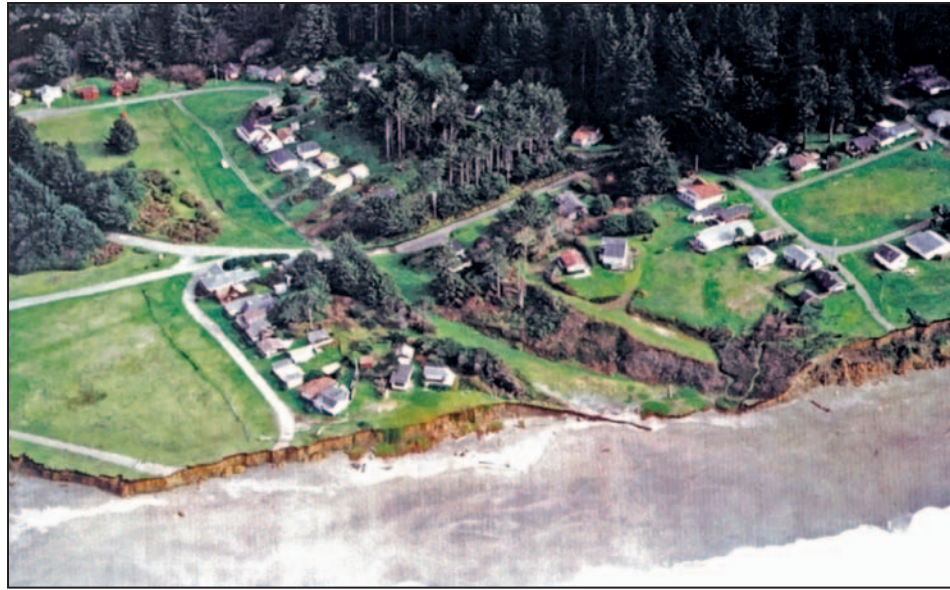
Figure 4-19. As buildings in this Humboldt County, CA, community are threatened by bluff erosion along the Pacific Ocean, they are moved to other sites on the jointly owned parcel
