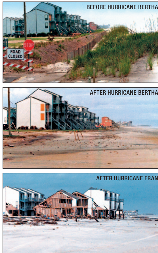
Figure 4-6. Cumulative effects of storms occurring within a short period at one housing development in Jacksonville, NC, July–September 1996
