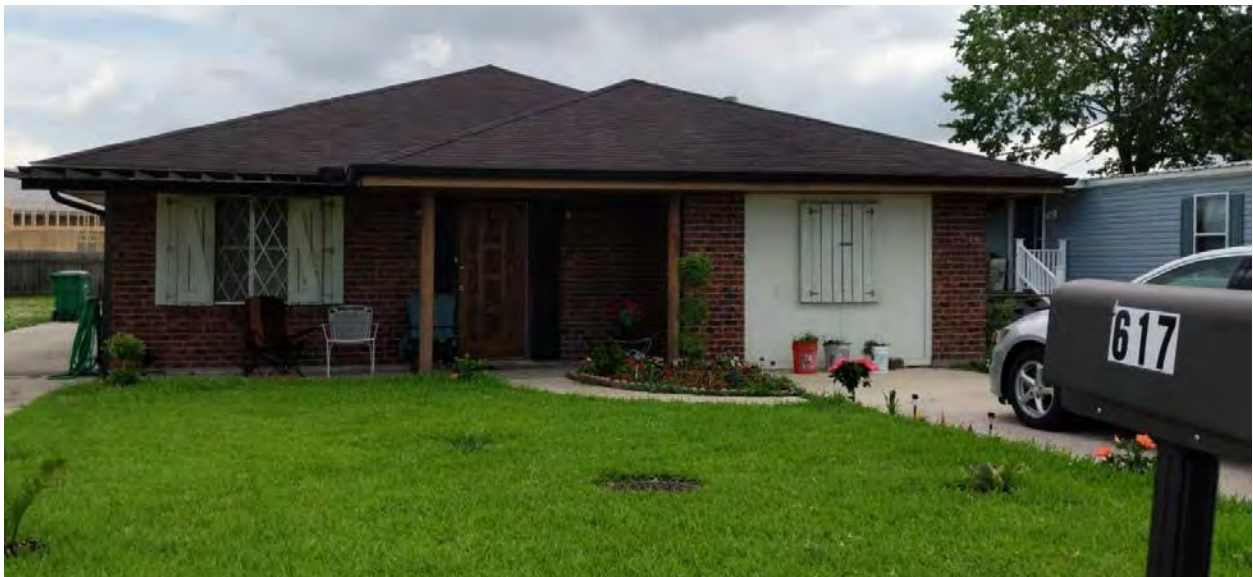
Figure 1- 9 Example Slab on Grade property in Rep Loss Area
