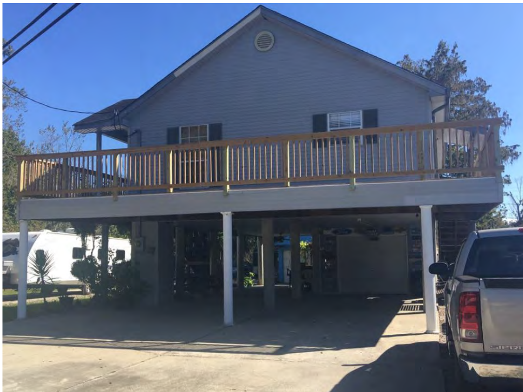
Figure 2-10 Example elevated property in study area
