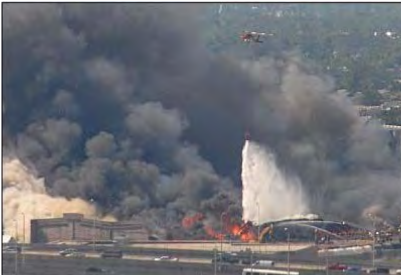
Figure D-13 Warehouse Fire (Source: FEMA)
