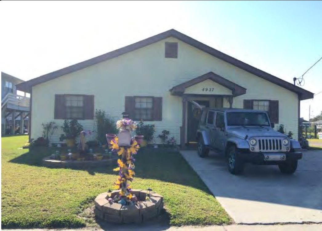
Figure 2-9 Example slab on grade property in study area
